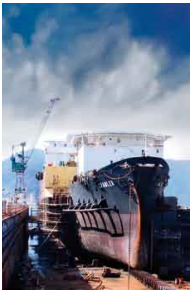
A dry dock at Palermo Shipyard
