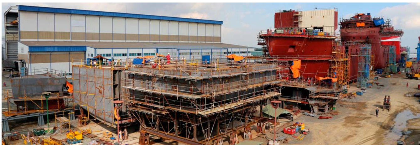
Vard Vung Tau, a fully-integrated facility capable of undertaking the entire process of shipbuilding.
