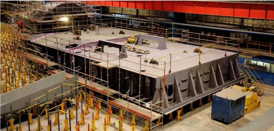
Production of hull sections for FINCANTIERI at Vard Tulcea.
