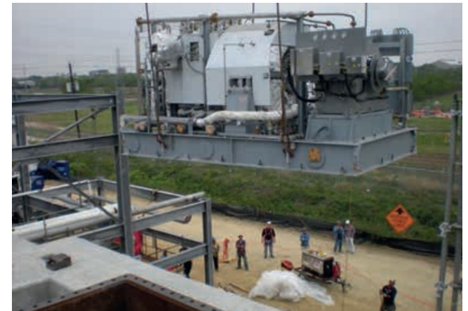
— STG set erection activities on site in USA
